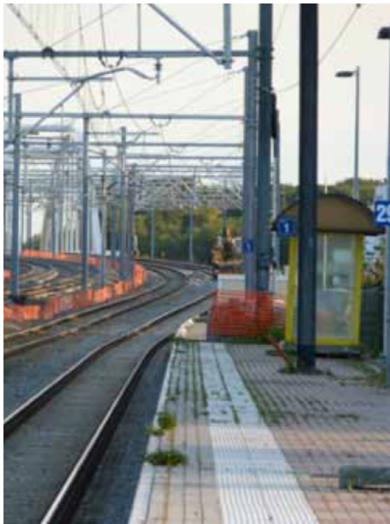
Figure 6 Simple plastic mesh Fences in Duffel Belgium
