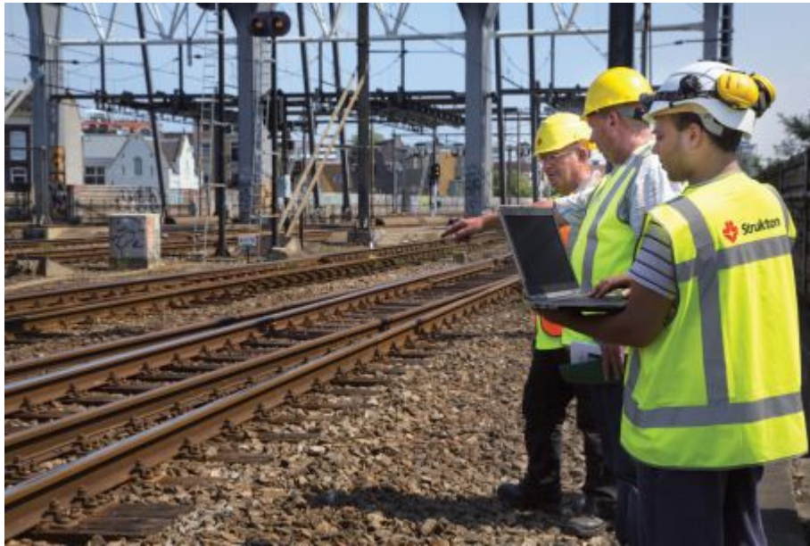
Figure 4 Track inspection near bridge using a form of SCWS (photo courtesy of ProRail)
