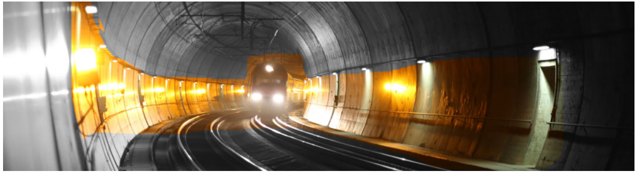
Figure 1 Fixed warning system in a tunnel
